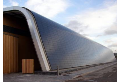
LSBIPV – OptIC Centre, Wales
