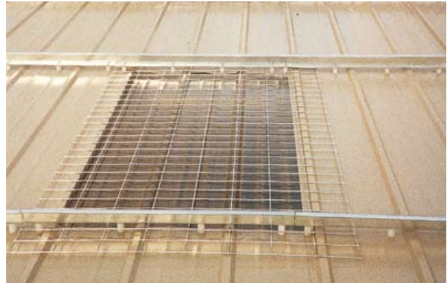
Figure 47 Galvanised mesh reinforcement between sheets of twin-skin roof light
