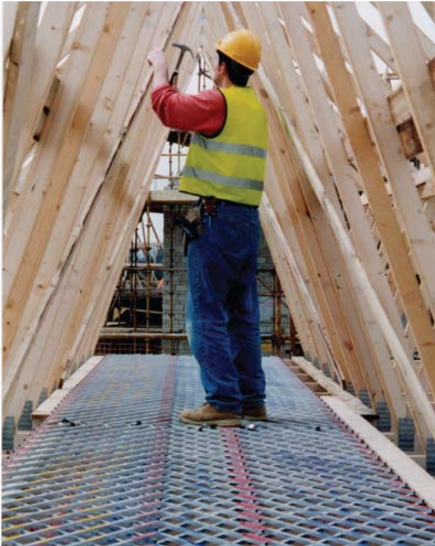
Figure 15(a) Decking system that provides a working platform in the roof eaves (Image courtesy of Oxford Safety Components Ltd)
