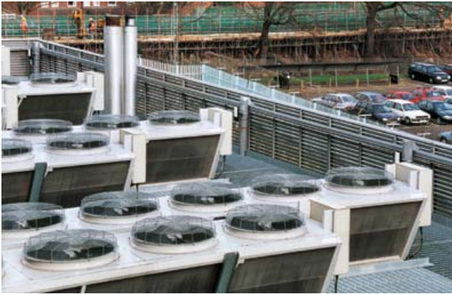
Figure 44 Parapet edge protection included as an integral design feature
