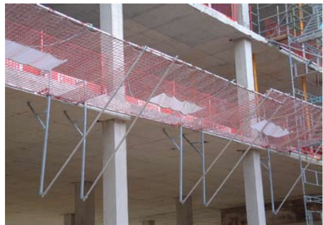
Figure 38(b) Debris netting (Image courtesy of Combisafe)
