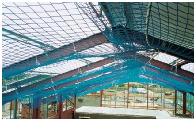
Figure 37 Use of safety nets during industrial roof work
