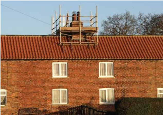
Figure 27 A traditional chimney scaffold
