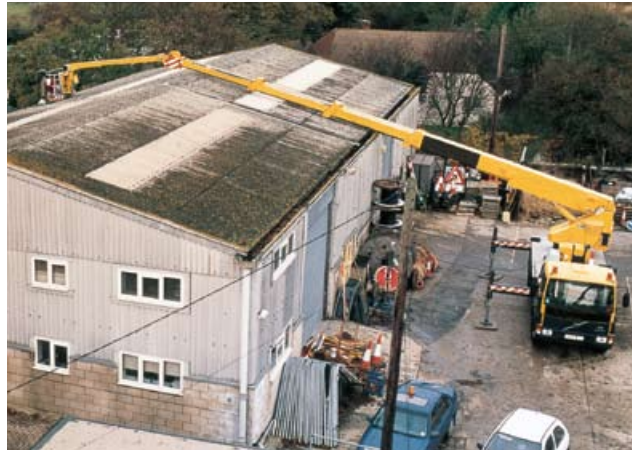
Figure 12 Powered access for inspecting a large fragile roof
