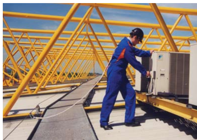
Figure 17 Work restraint harness used during short-term inspection on a flat roof (Image courtesy of Uniline Safety)
