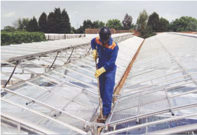
Figure 13 Valley walker used during gutter cleaning
