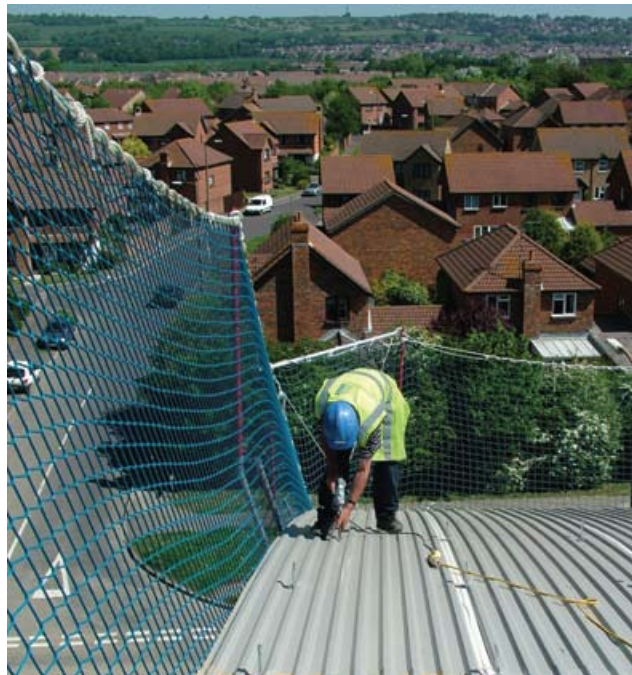
Figure 36 Netting capable of providing edge protection
