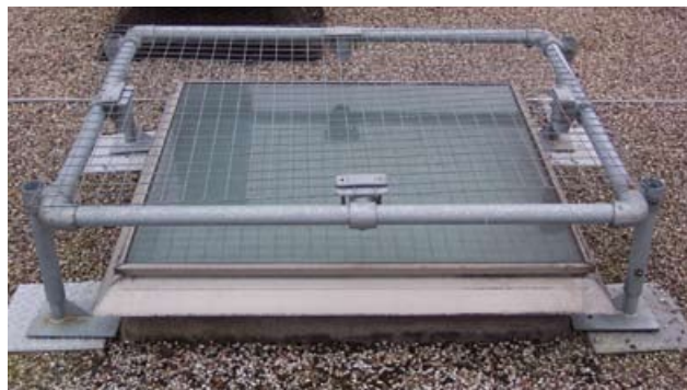
Figure 48 Covers can be fitted to existing roofs or included as part of the design (Image courtesy of Safesite)
