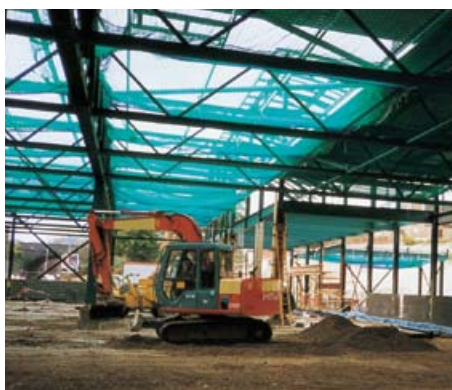
Figure 8 Debris netting used in addition to safety netting may enable work to be carried out safely below roof workers
