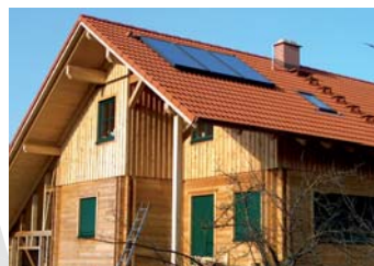
tecSol on inclined roof
