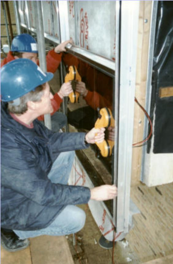
**Positioning modules using suction lifters**
