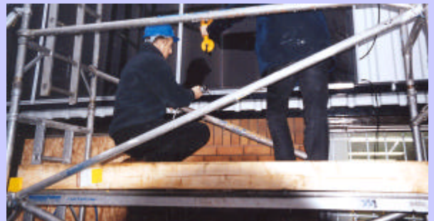
Working from scaffolding
