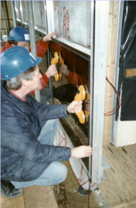
Positioning modules using suction lifters
