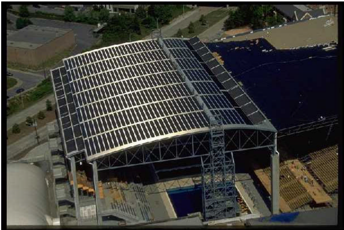
Aerial view of PV roof at GTAC, Georgia, USA
